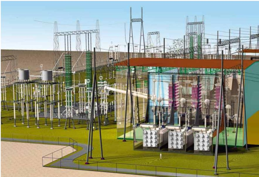
**7** An HVDC converter station with four power blocks – the configuration is chosen to minimize the effects of individual component failures
